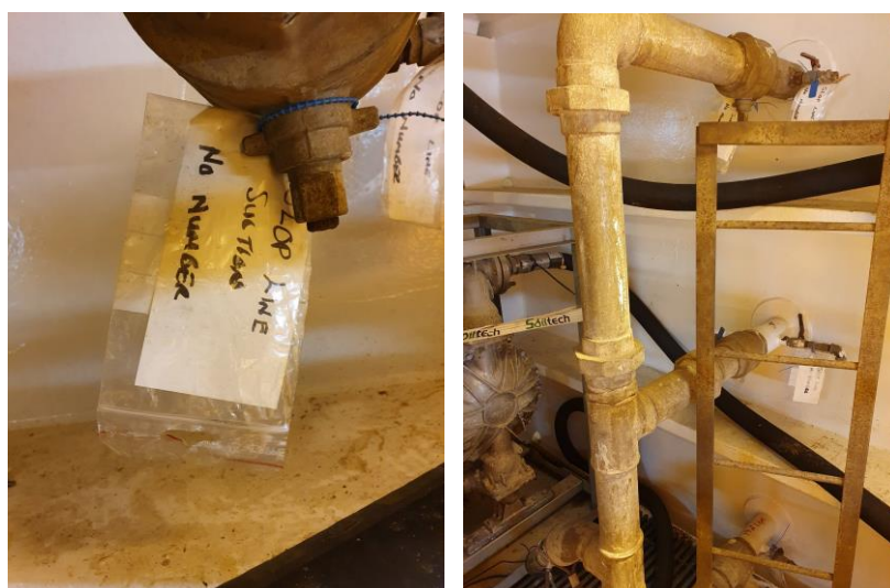
Figure 4-7: Insufficient labelling of pipes in pump room
