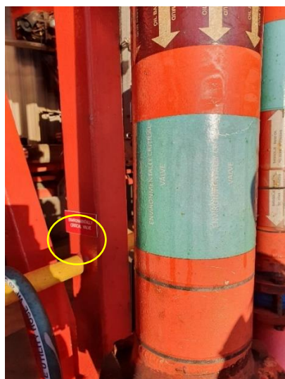
Figure 4-3: Green labels on pipes closed with environmental critical valves. These valves are also marked with red tags (yellow circle)
