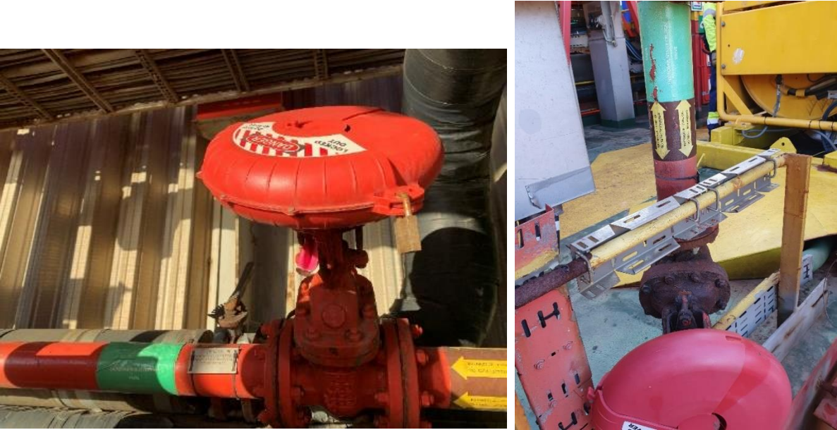
Figure 4-4: Environmental Critical Valves for Fuel oil with green labels, starboard side to the left and port side to the right
