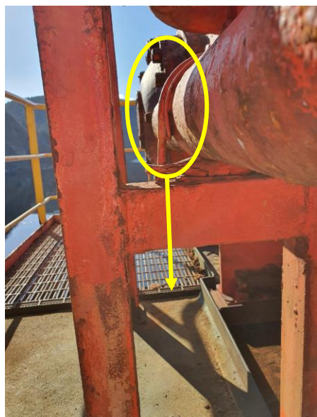
Figure 4-8: Bundling insufficient at anchor winch #3
